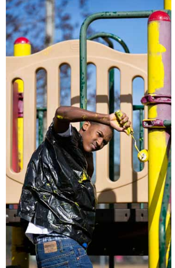
Kevin Baxter, a senior at Scott's Branch, applies a fresh coat of paint to playground equipment at Wausau Park.
